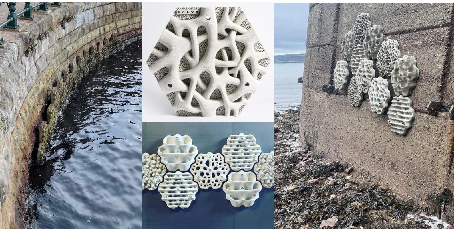
*Two middle images taken from the VOLVO's living sea wall project and used to show the up-close 3D geometry of each tile, which mimics the structural complexity of native mangrove roots.
